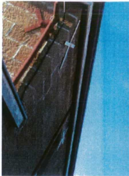
Photo 1.9 East Wall Oct 2005
