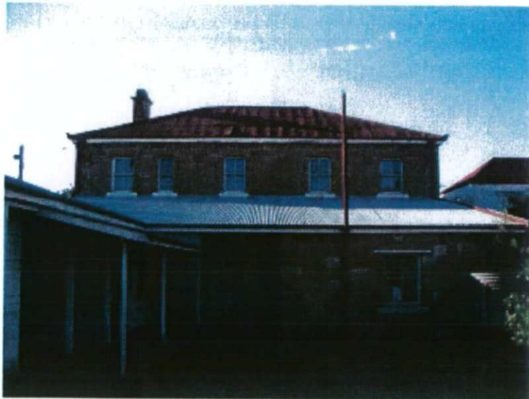
Photo 1.3 Rear Newer Building from rear yard June 2007
