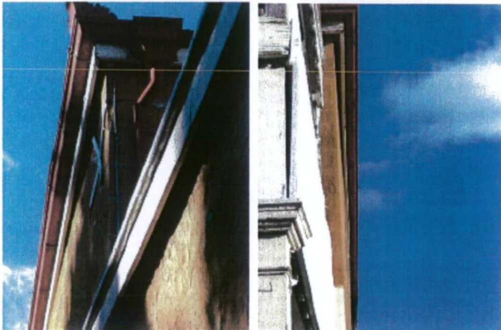
Photo 2.3 2.4 West wall existing condition
