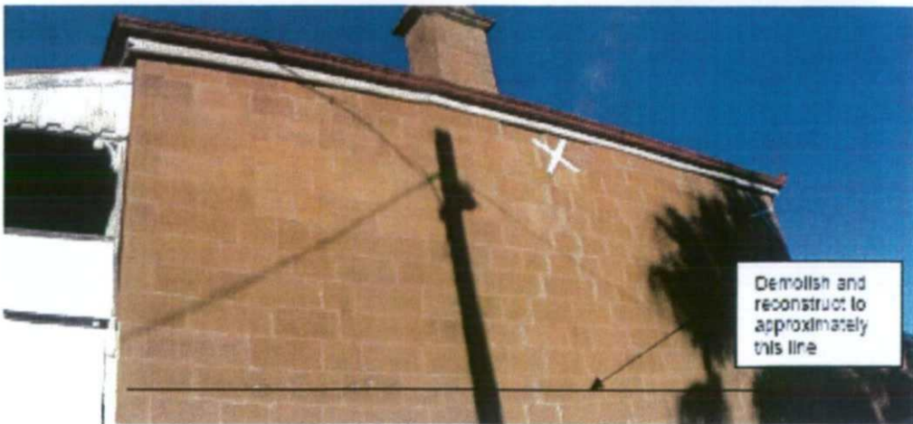
Photo 2.5 West wall reconstruction
